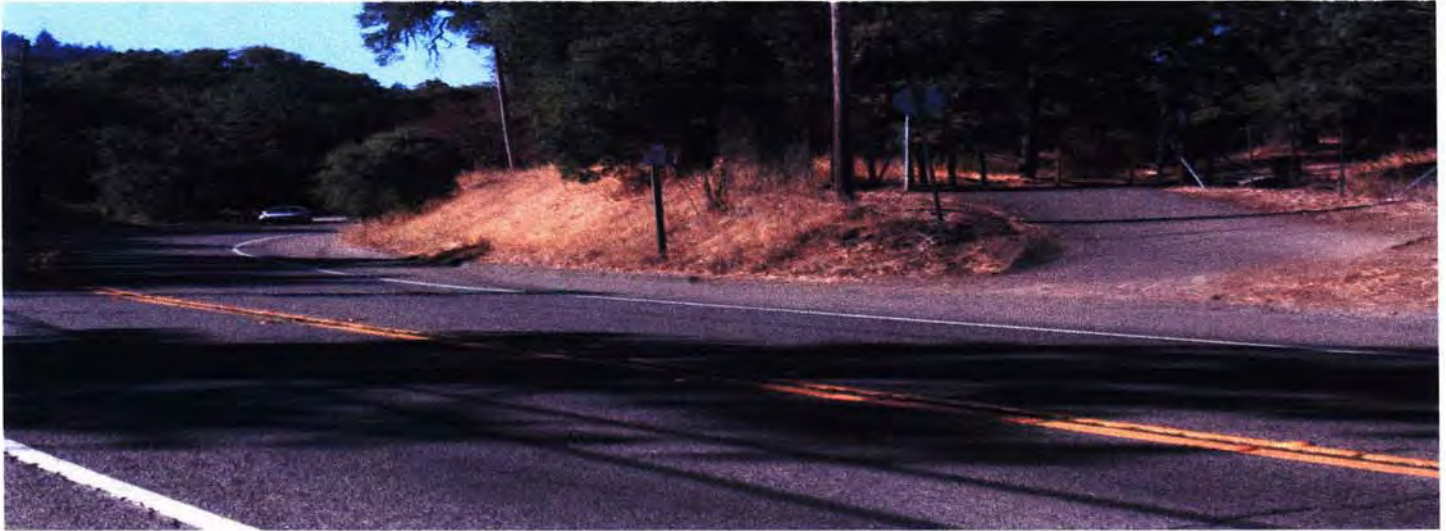
Arnold Drive entrance to Regional Park & bike path to Dunbar/Glen Ellen. Note curve & high speeds.
