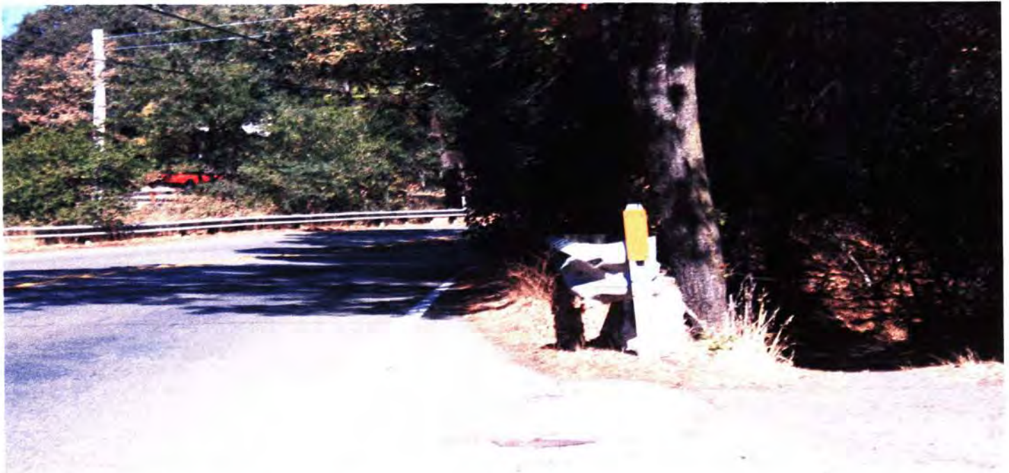
Overgrown trees & grass on Arnold north of Jack London Village.
