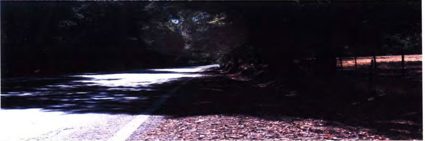
Flat part of Arnold Drive where bike lane could be made wider
